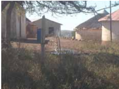
Figure 1.10.5: An illegal connection under construction discovered by our staff members in Phathane in uMfolozi
